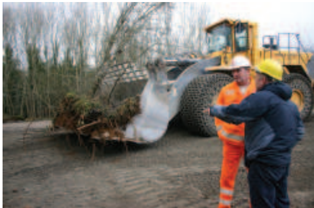
Fig. 4. Eight-tonne shovel picking up a 1m slice of soil and woodland for translocation to nursery bunds and abandoned faces
