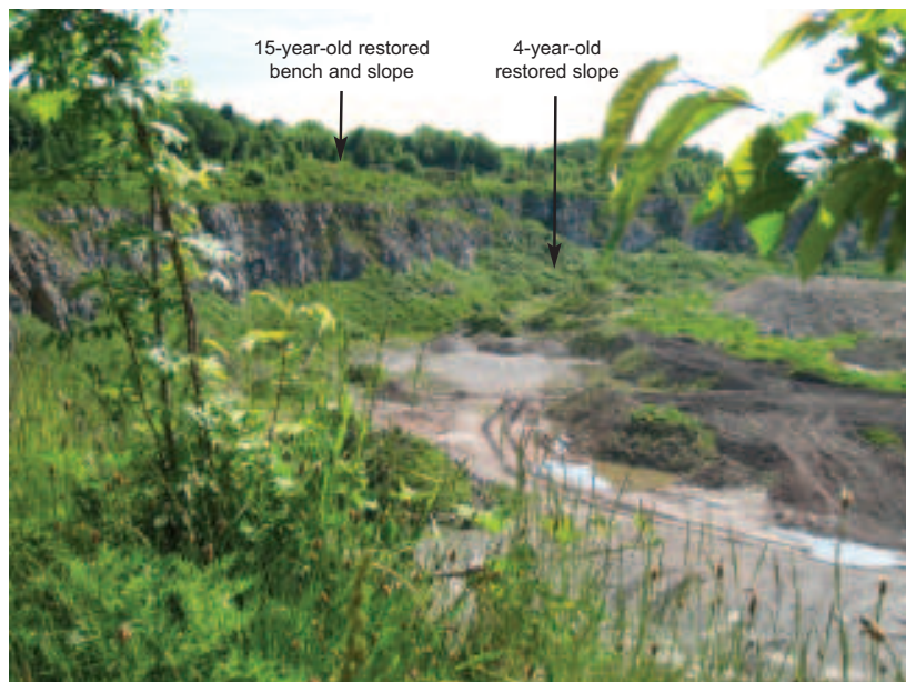
Fig. 2. View of 15- and four-year old restored slopes on the southern limit of the working at Cefn Mawr
